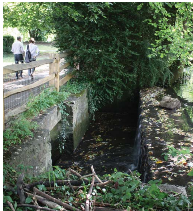
Sluice within the central lake
