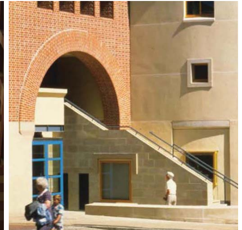
Epping Forest Civic Offices
