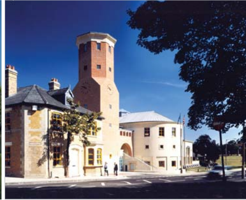
Epping Forest Civic Offices
