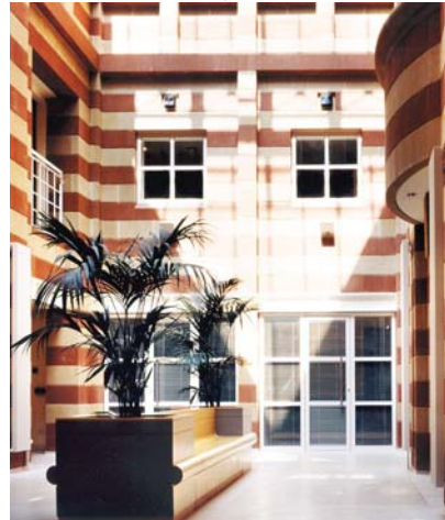
Epping Forest Civic Offices
