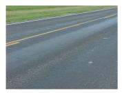
The ability of a road surface to resist vehicles skidding reduces over a period of time due to the wearing and polishing effect of the many thousands of vehicles that pass over it. In the case of bituminous roads, it may also be caused by heat damage leading to higher levels of bitumen on the surface. Either through
