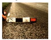
When subjected to continuous high levels of traffic bituminous roads develop rutting in wheel track areas. The use of the road by traffic displaces the surfacing, and sometimes the materials within the road structure, by creating an uneven running surface that can, if severe, present a hazard. Although some materials used in more recent years are less prone to rutting, it still does occur on roads that carry high numbers of HGVs.
