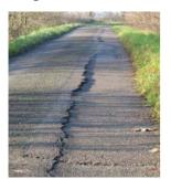
Edge deterioration can be caused by several factors and generally occurs on un-kerbed rural lanes. It can take a number of forms such as deformation, potholes, cracking or a combination of all.
