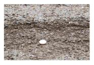
held together by a binding material, originally tar, but now bitumen as stated above (hence the term 'Tar-mac'). This form of road construction was developed by John Loudon McAdam in the 1820's and over the subsequent years there have been many innovations in materials but the principle remains the same.
