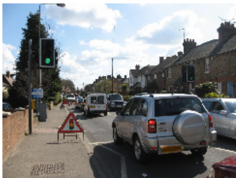
Photo 19 - Partly obscured 30mph speed limit sign
