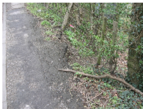
Photo 80 - Footpath subsiding
