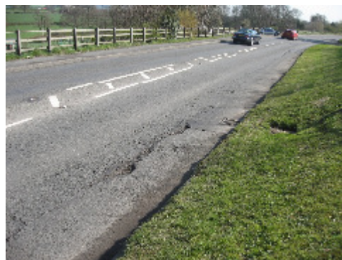
Photo 45 - Carriageway deteriorating
