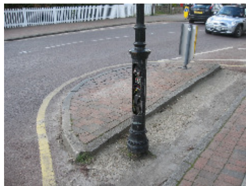
Photo 32 - Missing lamp column door
