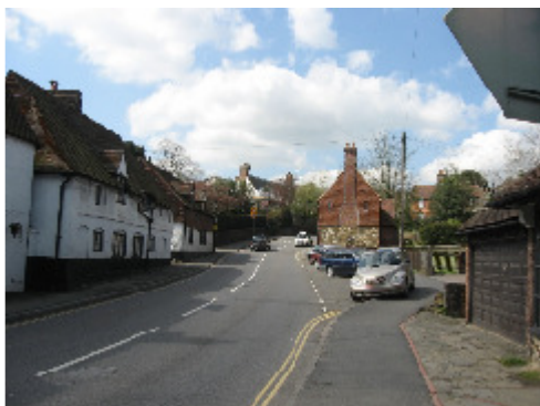
Photo 62 - Lay-by lines are worn and a section unpainted
