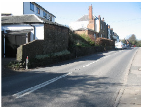
Photo 13 - Road marker posts coated in grime
