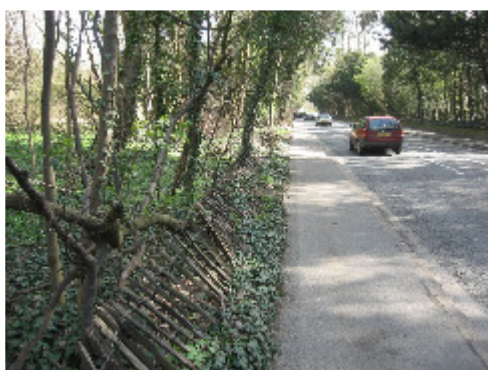
Photo 25 - Wooden fence is in a poor condition
