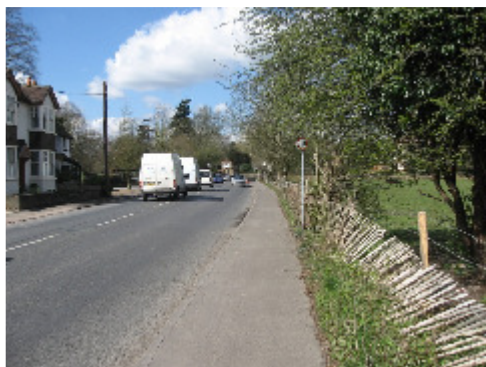
Photo 21 - The wooden fence is in a poor condition and 30mph speed limit sign partly obscured by vegetation
