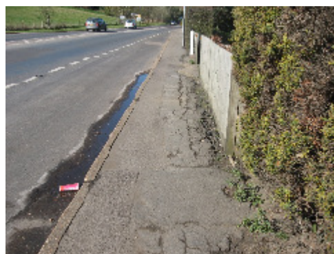
Photo 11 - Edge of carriageway
