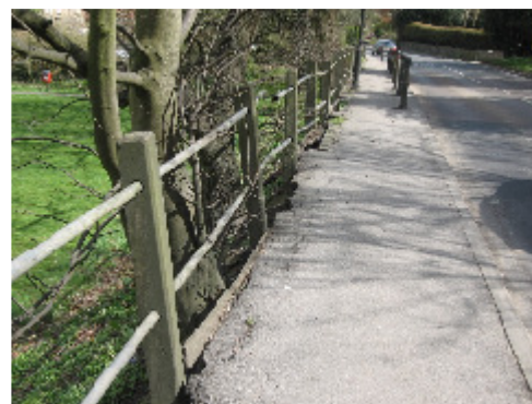
Photo 41 - Footpath subsiding
