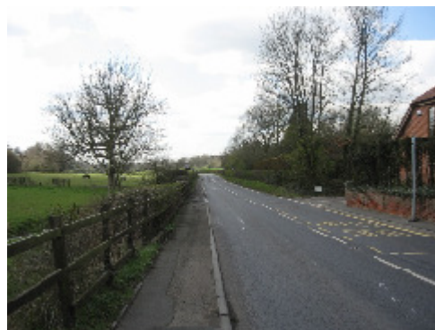
Photo 75 - Footpath is in a poor condition
