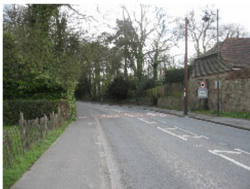
Photo 27 - Obscured 30mph speed limit sign
