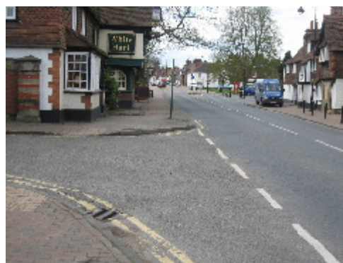
Photo 30 - There is a redundant pole
