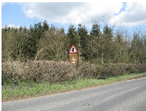
Photo 77 - No carriageway edge road markings and an outdated tourist sign
