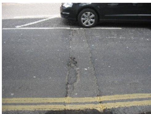
Photo 67 - Carriageway deteriorating
