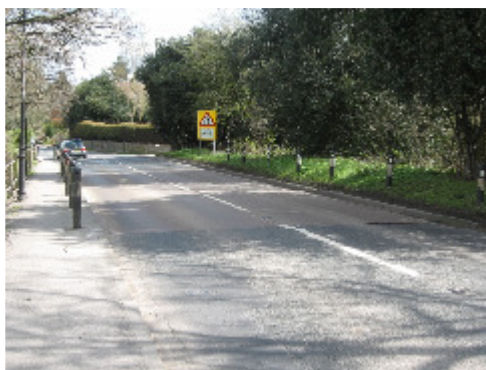
Photo 40 - Road marker posts are coated in grime
