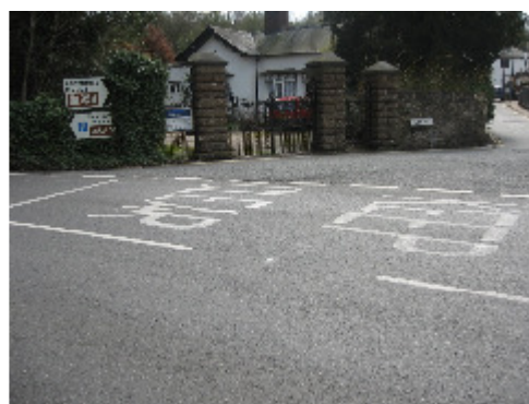
Photo 61 - Pothole in junction interface and partly obscured sign
