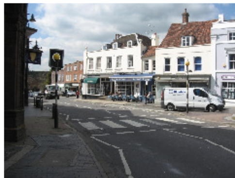
Photo 66 - Road markings are worn
