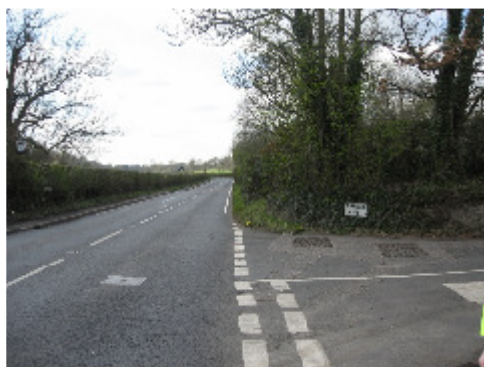
Photo 76 - The view to exit Farley Lane is severely restricted
